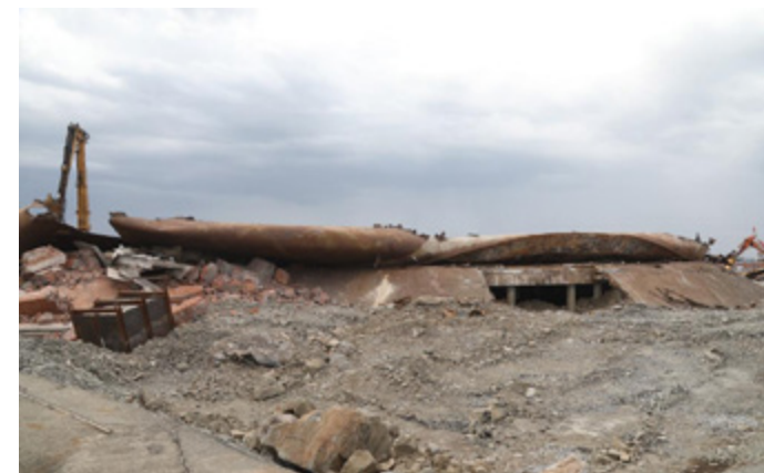
Fig. Disassembly of damaged tank No. 5
