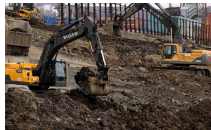
Fig. Contaminated soil collected and removed from the spillage area
