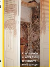
Warping floors and discoloration of walls and ceilings can be indications of moisture problems. Condensation on windows or walls is also an important indication, but it can sometimes be caused by an indoor combustion problem! Have fuel-burning appliances routinely inspected by your local utility or a professional heating contractor.
